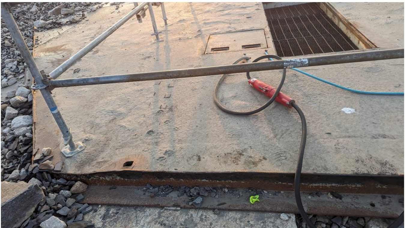
Figure 5: Survey control point (yellow) bolt near IOL dock
